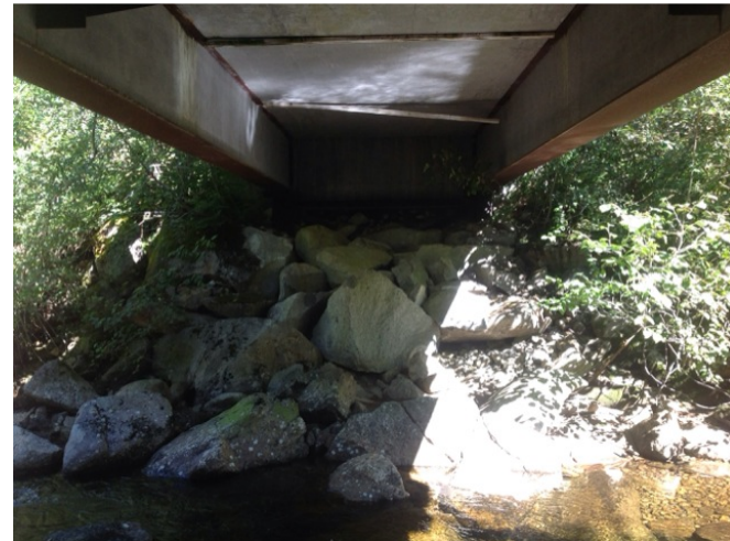
Left Bank Abutment when facing downstream
