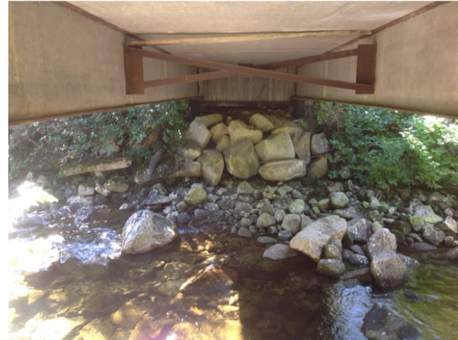
Right Bank Abutment when facing downstream
