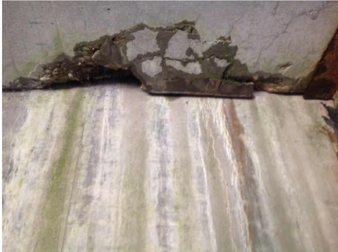
under deck panel 1
